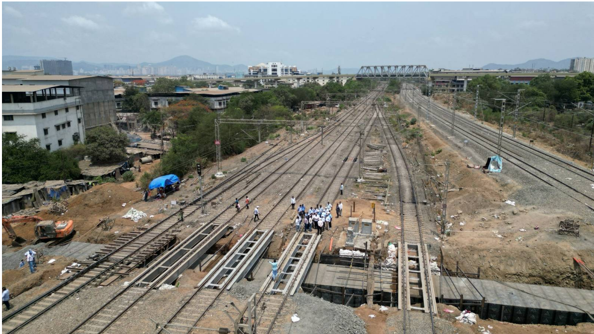
Track and civil works executed within an operating railway corridor.
