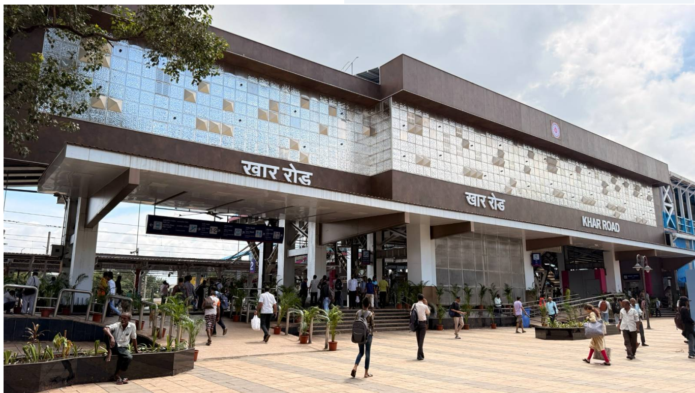
Station infrastructure - Khar Road.
